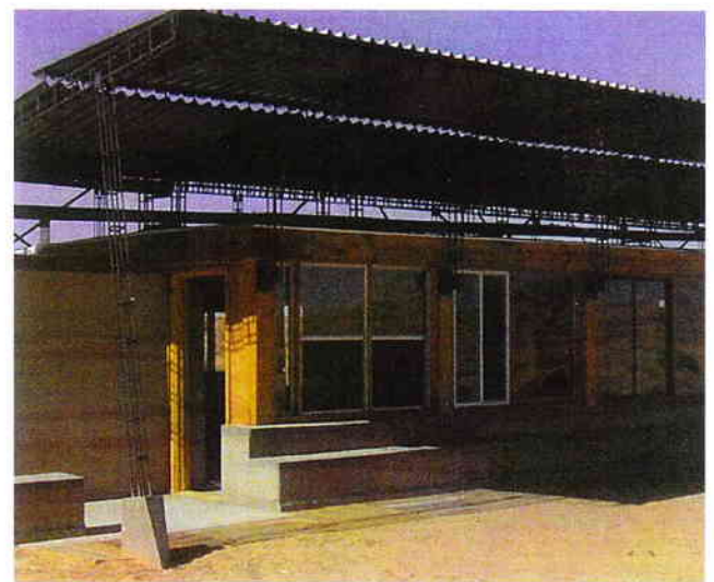
The award-winning Rosie Joe House in Bluff, Utah, designed and built by U of U graduate students in architecture.
