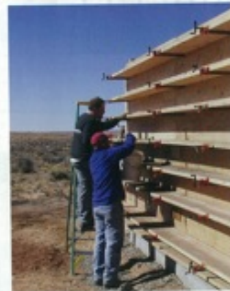
Clockwise from top left: Timber wall system made of rammed earth for the Sweet Caroline house (2006); Hank Louis, the founder of DesignbuildUP, tests SPF panel of a wall for Studio 23; Living space and central fire place of Sweet Caroline house (2006); Students build frame for a rammed earth wall for a passive solar system for the Rose Joe House.
